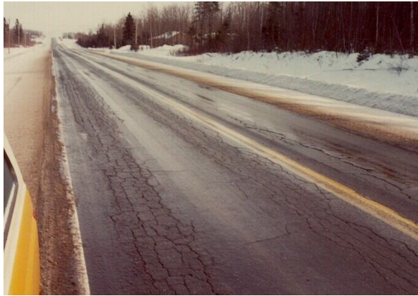
Figure A2-1 : Example of pavement damage due to frost-thaw effects
